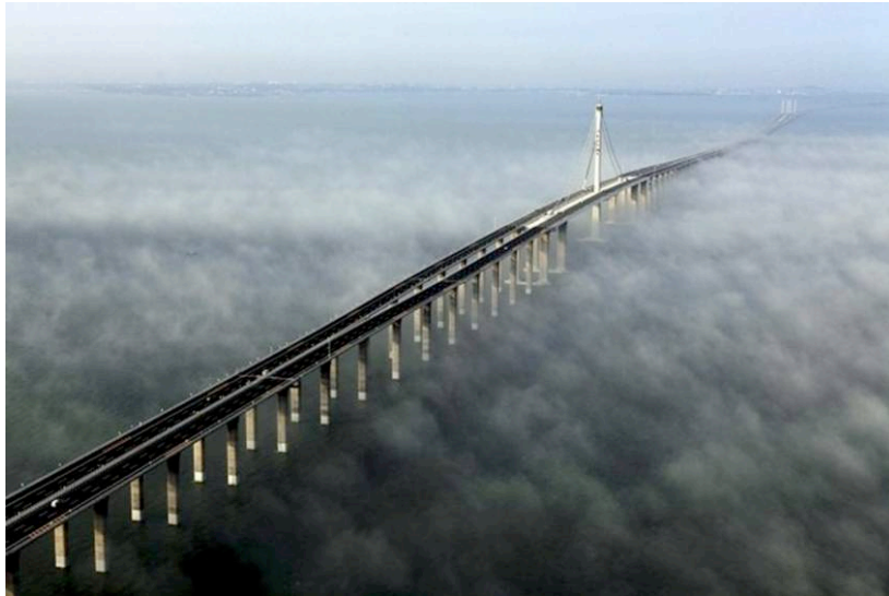
航拍胶州湾跨海大桥 Qingdao Jiaozhou Bay Bridge
